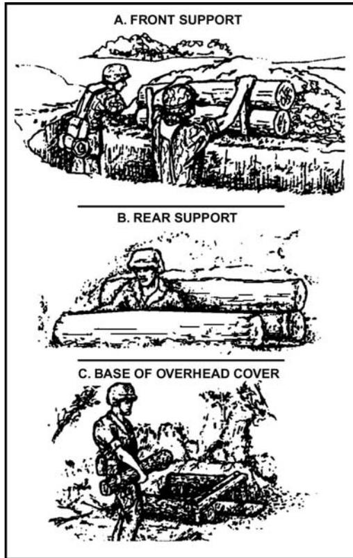
Figure 071-326-5703-5. Constructing overhead cover
